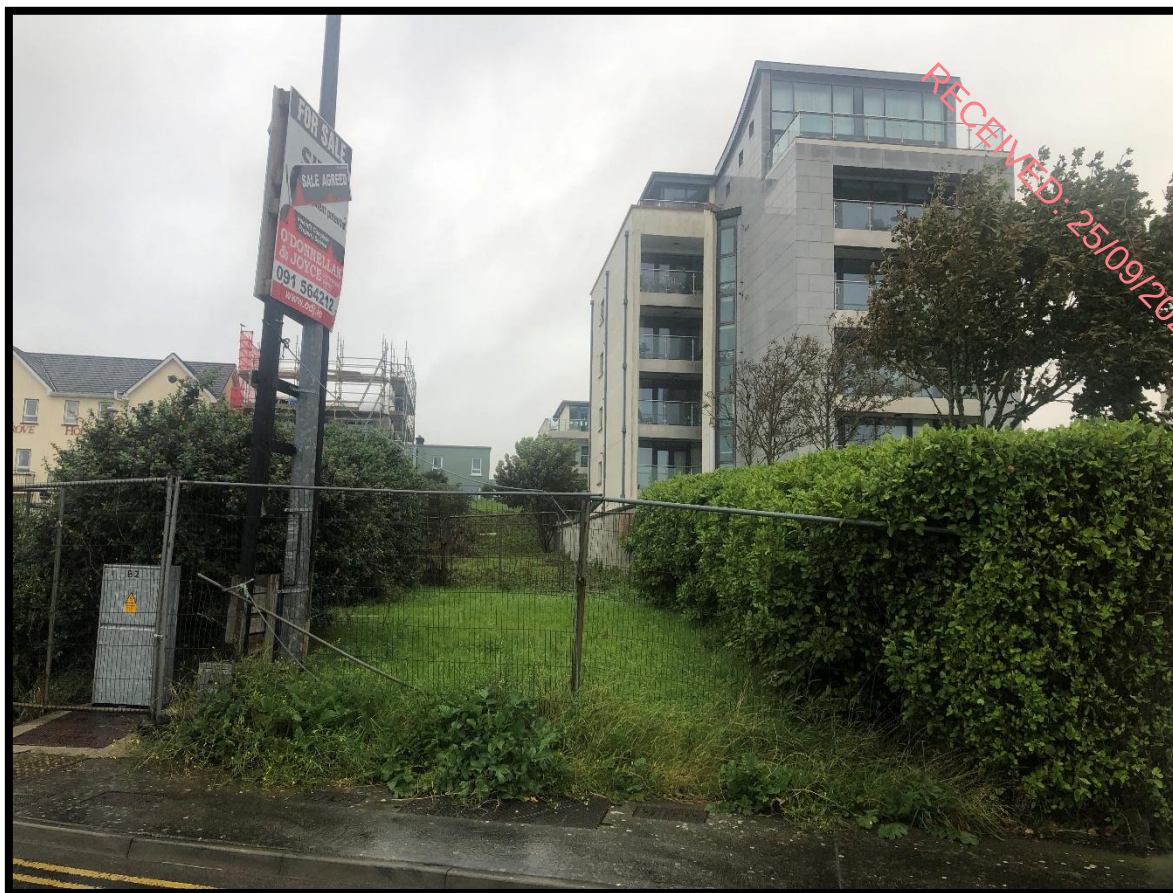
Plate 4.1 Looking north from the south of the site
